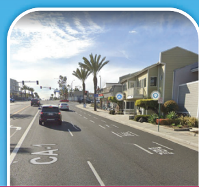
NORTHBOUND PCH AT GOLDEN LANTERN (BEFORE INTERSECTION)
